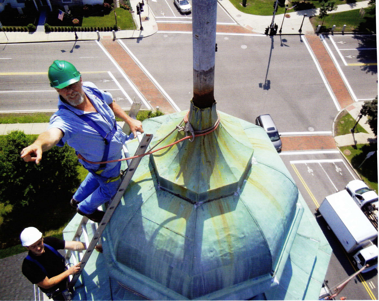
Photos by BOB LEVESQUE of American Steeple and Tower Company
